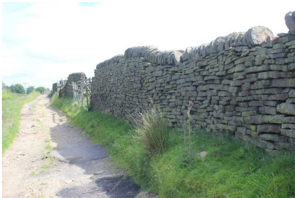
Dry stone walling showing half round tooled copings
