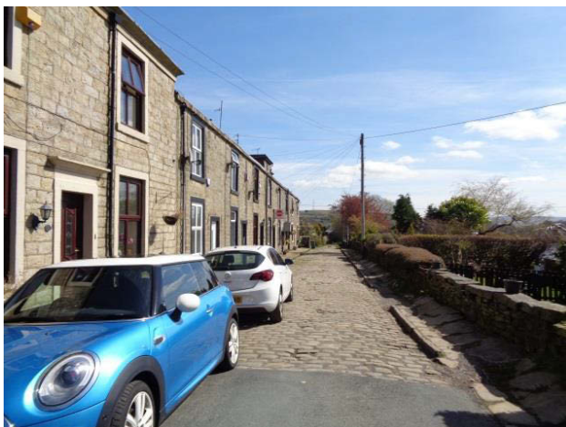
Terraces on Smallshaw Road
