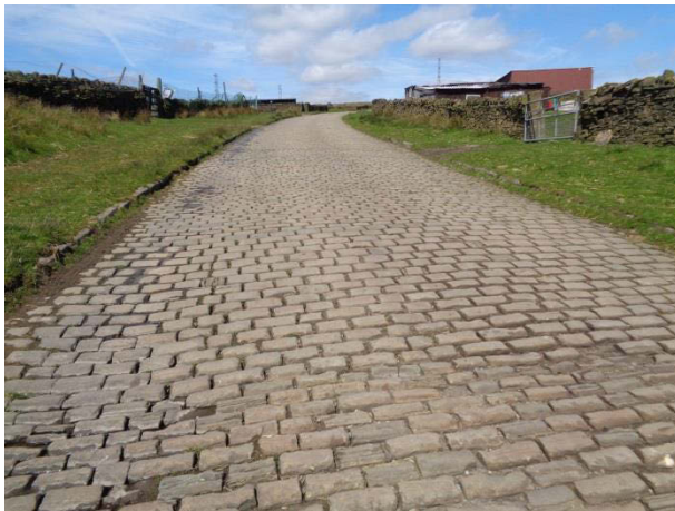
Paving on historic Cotton Famine Road
