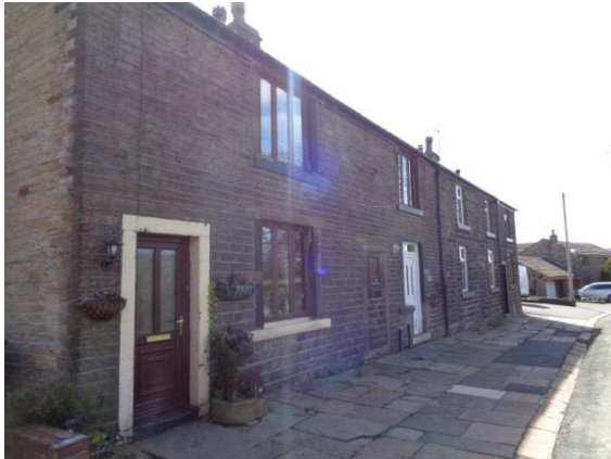
Wide pavements built using local stone flags
