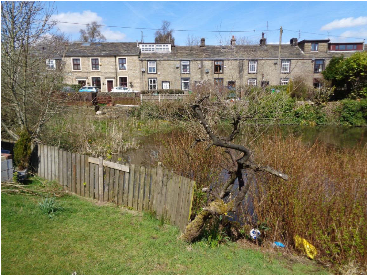
Housing on Smallshaw Road, the reservoir and gardens demonstrate the mix of spaces
