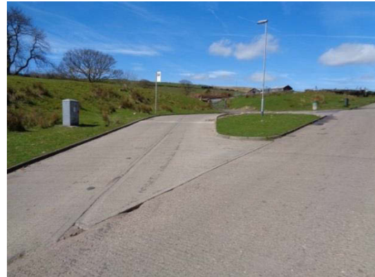
Construction of the bus turning circle in 1982 and the circle in 2016
